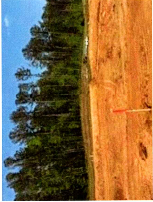
Eroded Area C+200 to D+150 Exposed Liner
